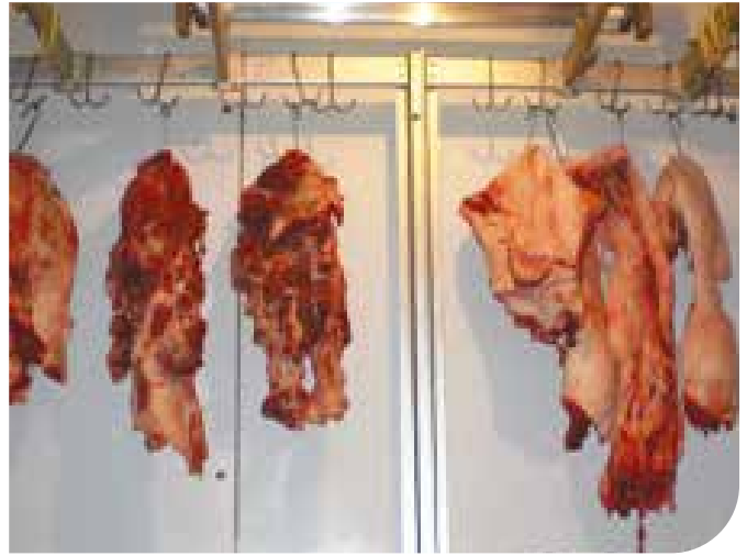
Forced Air Tunnel
